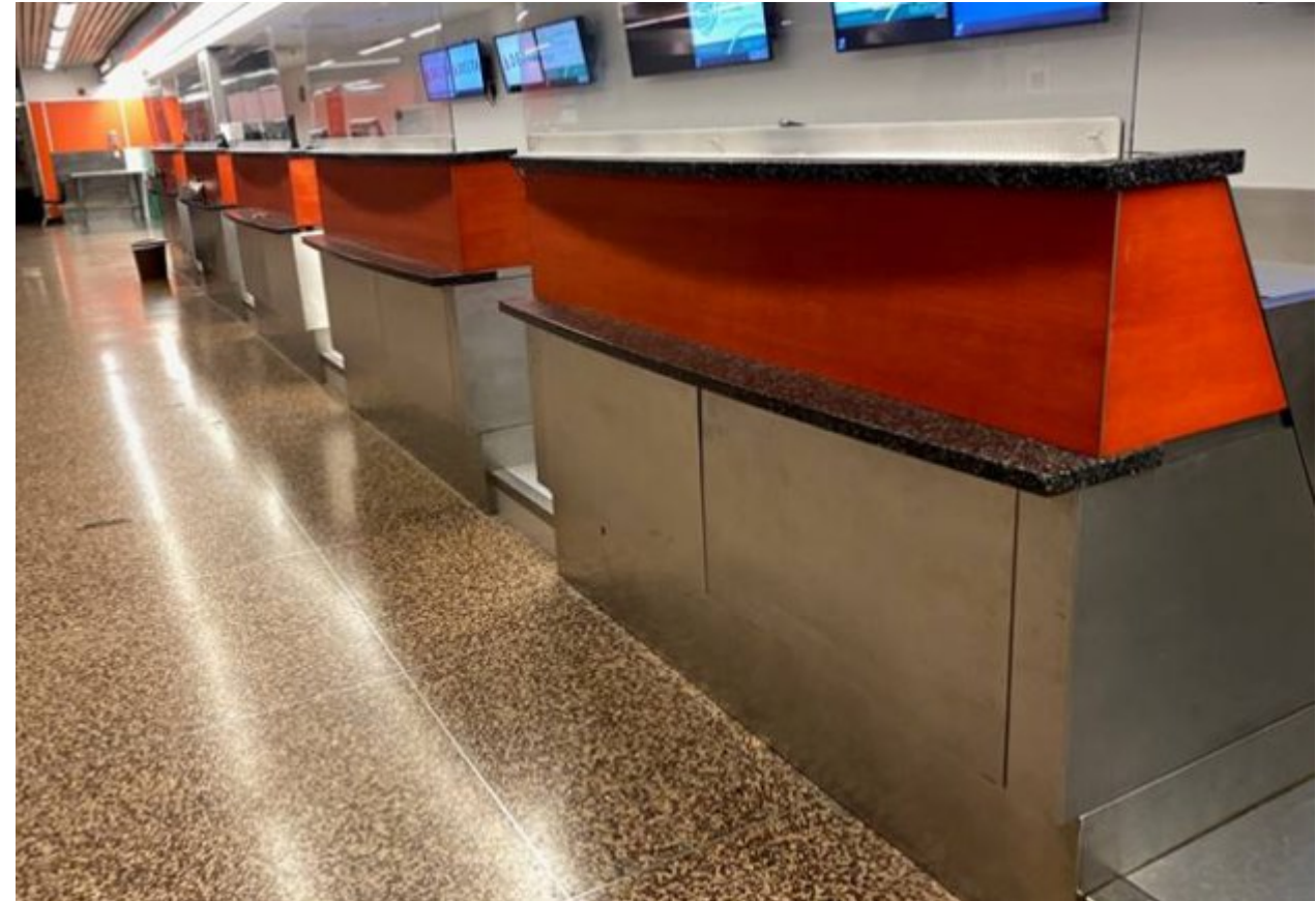
Replacement Ticket Counters
